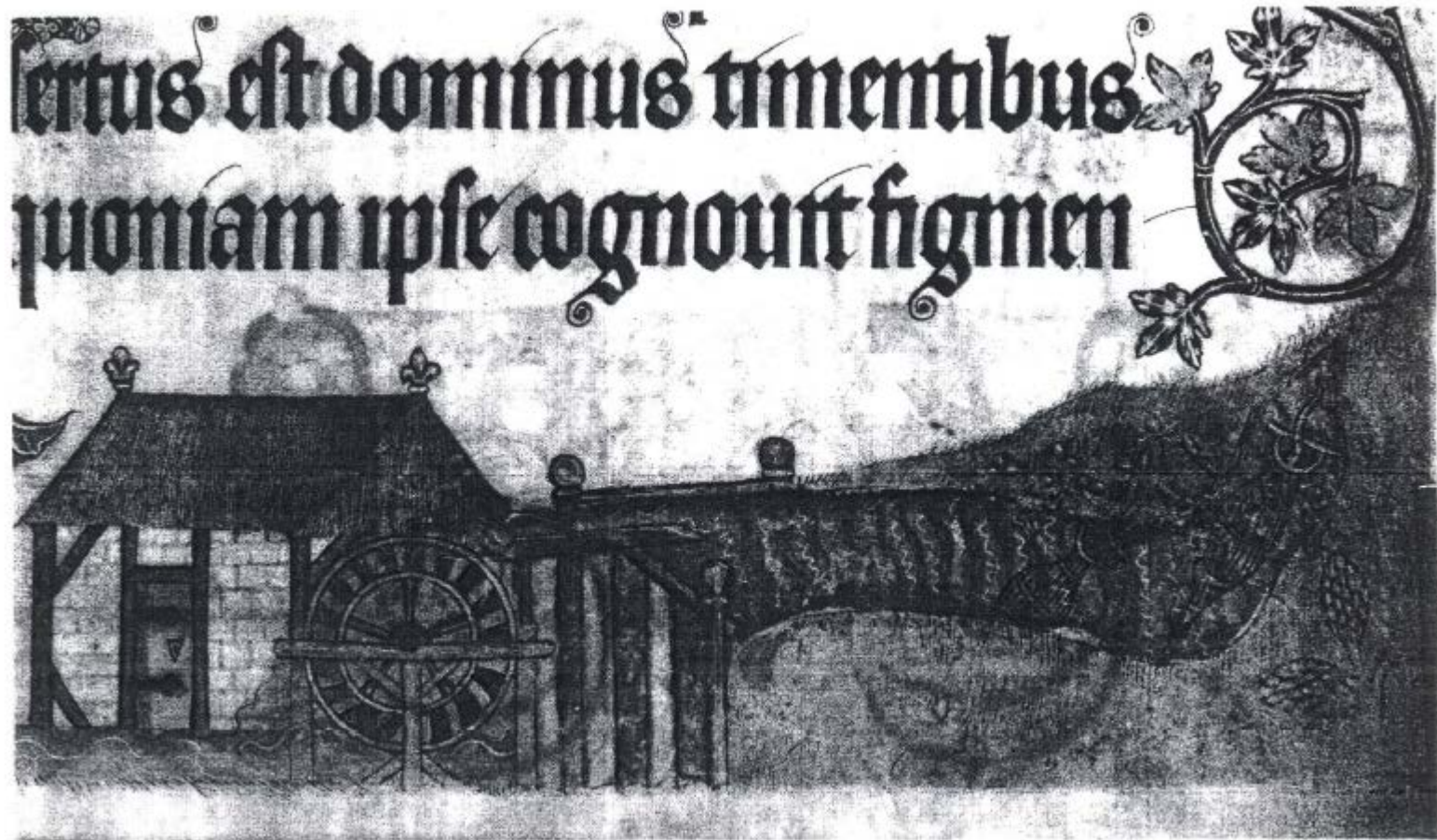
Plate 3 A fourteenth-century watermill from the Luttrell Psalter (British Library Add. Ms. 42130 fo. 181). The mill-pool contains traps for eels and other fish. Reproduced by kind permission of the British Library.
