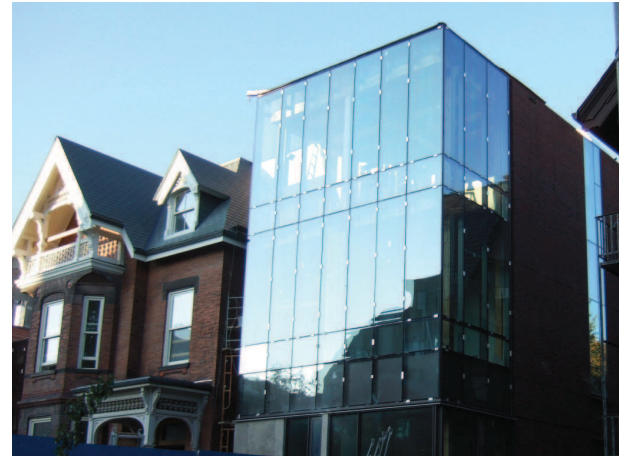
New Department of Economics building, photo as at October 30, 2008
