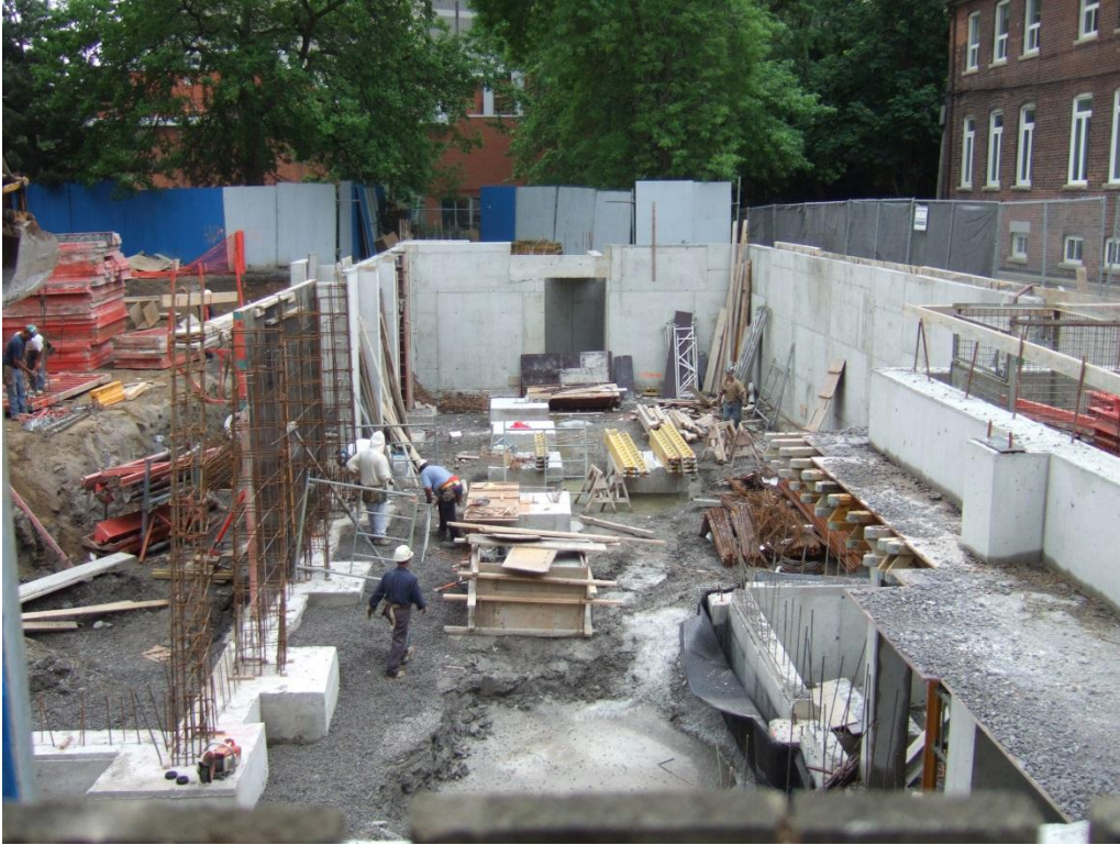
West Wing: Basement looking south 5 June, 2007
