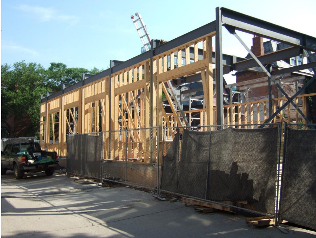
First floor conference rooms looking NE from bpnichol lane 9 July 2007
