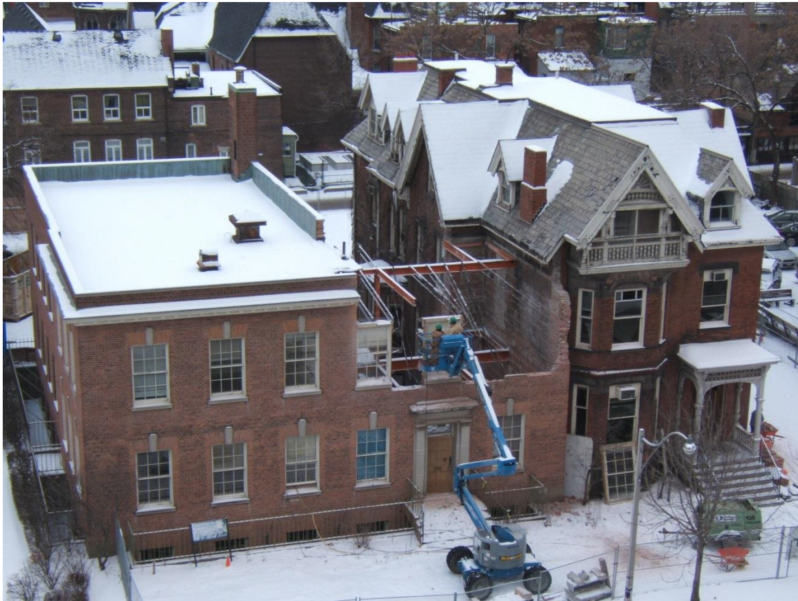
During demolition, from Rotman roof, 30 January 2007.
