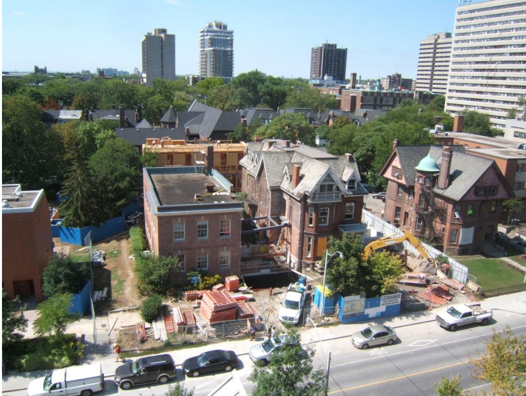
From Rotman Roof, 30 August 2007
