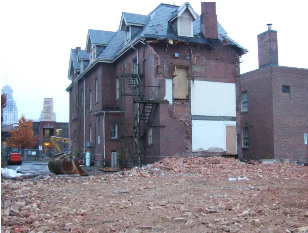
The original house after demolition of the 1920's addition and the coach house, looking east from the bp nichol laneway.
