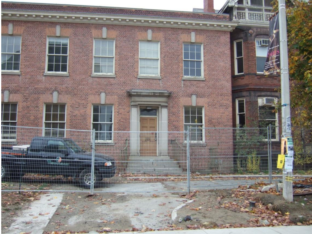
South Addition before demolition of connection
