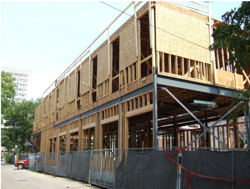
Conference rooms and offices looking NE from lane, 5 September 2007
