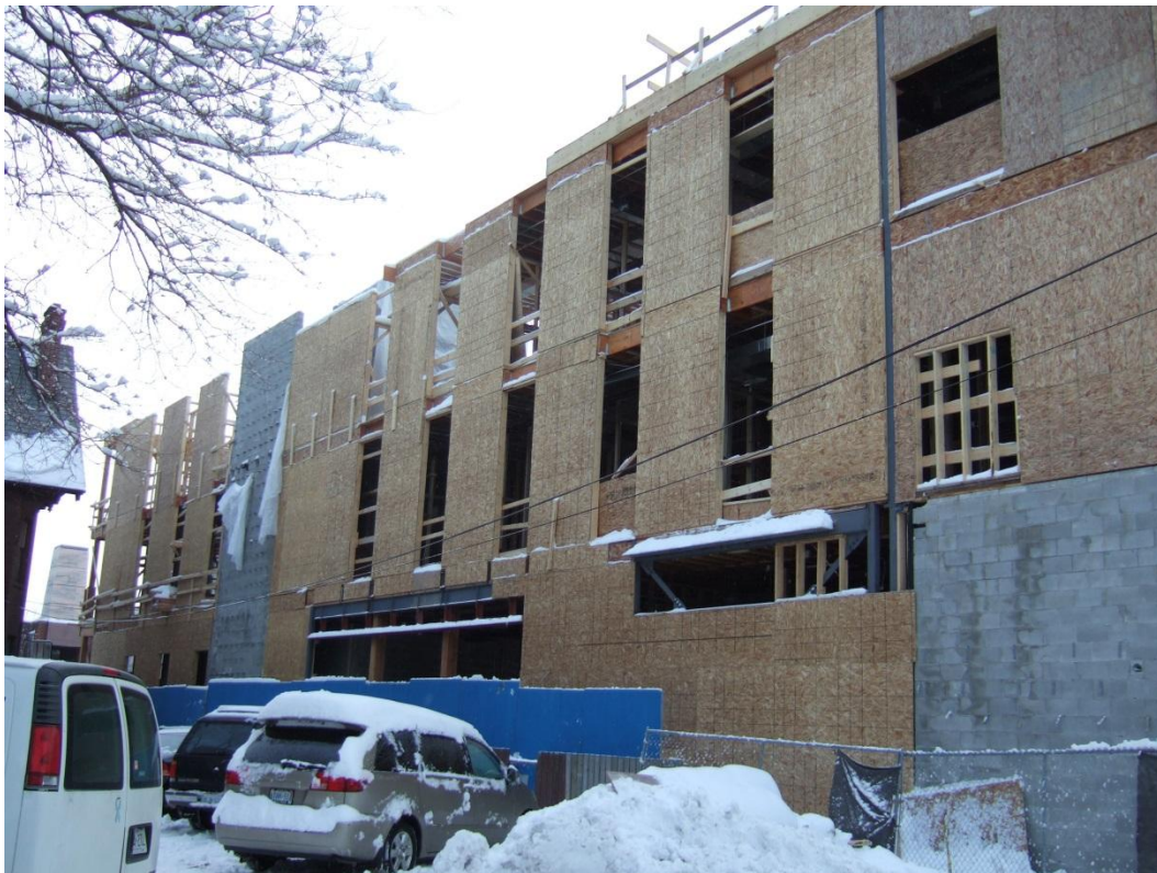
North Wing looking SE from fraternity parking lot, 8 February 2008
