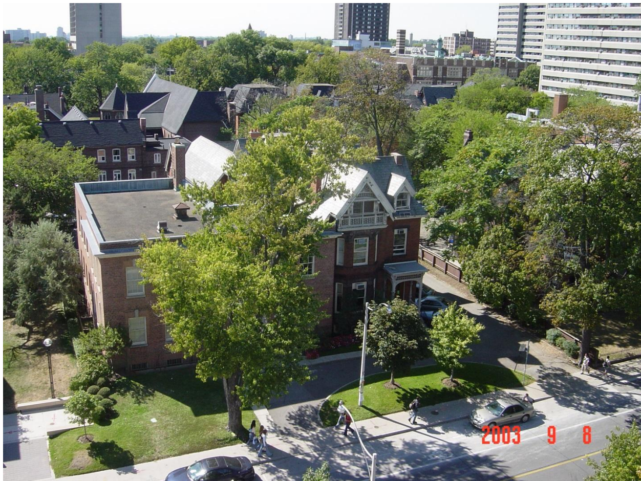
Economics building, 150 St. George Street, before renovation looking west from Rotman roof in September, 2003.
