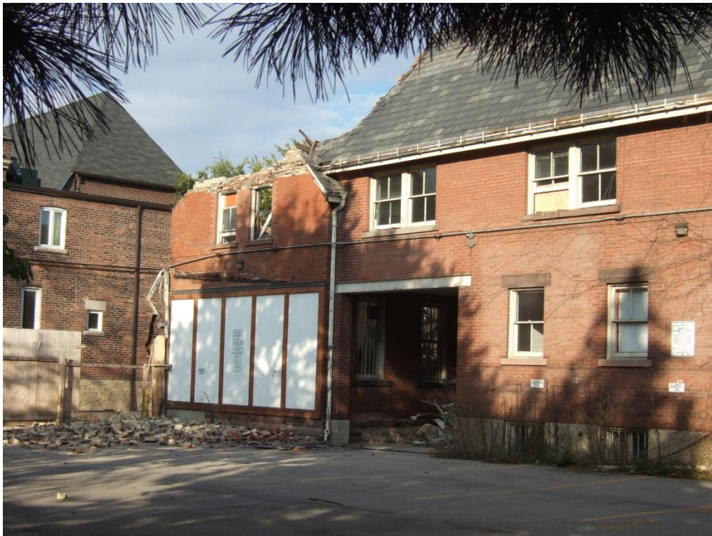
Coach House roof off looking NW.
