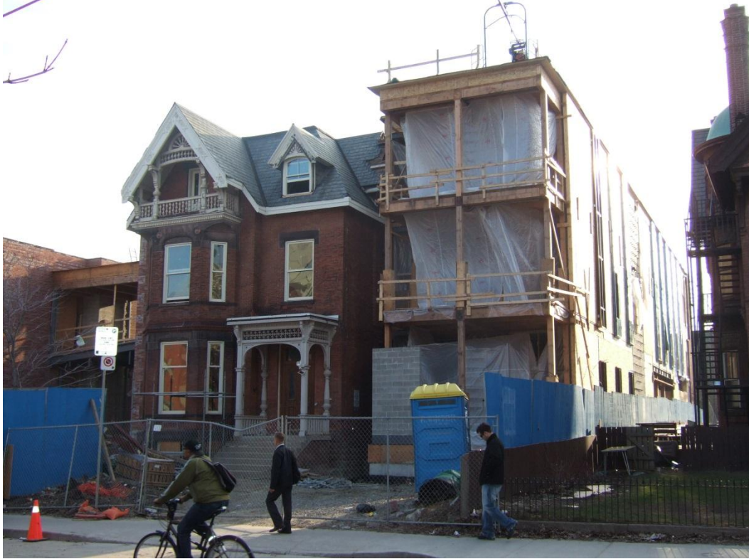
Front of house from St. George St., 8 April 2008.
