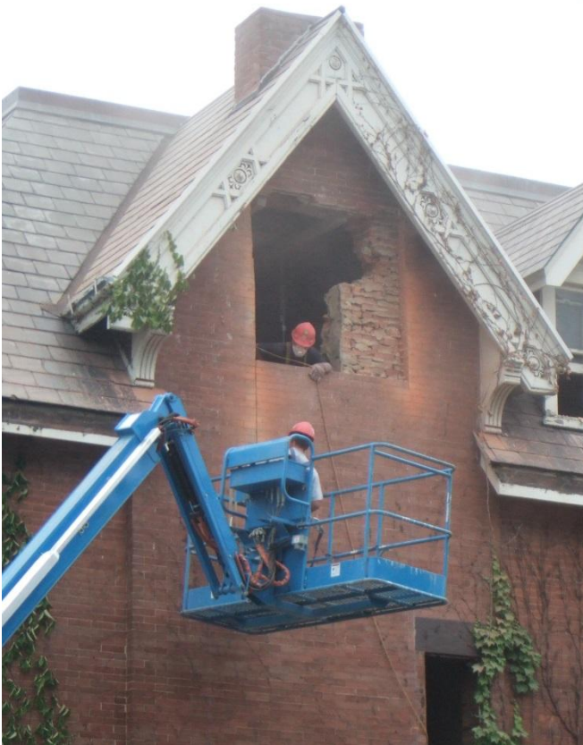
Crowther House, north side 19 June 2007: Cutting 3 rd floor passage through a chimney to new north wing.
