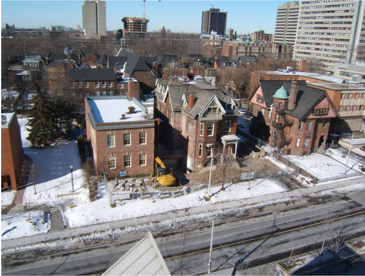
Demolition completed, ready to start construction, February, 2007.
